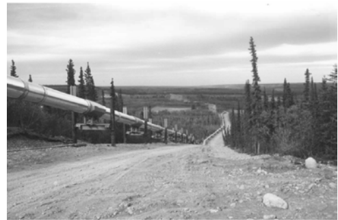
Figure 95. The Trans-Alaska Pipeline elevated above the ground on steel vertical-support members (VSMs) to prevent thawing... Photograph by O.J. Ferrians, Jr., September 1977...
