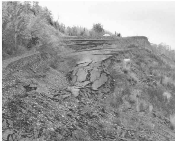
“Figure 92. View ( to the north) of abandoned road cut on Simpson Hill showing successive slumps that destroyed old road surface... Photograph by O.J. Ferrians, Jr., September 1977.
